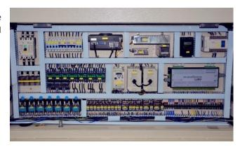
PLC controller Industrial PC in combination with an onboard UPS form a stable, safe and efficient controlling system.
