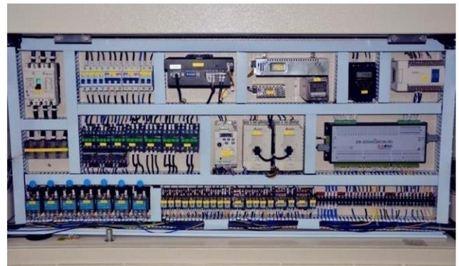
PLC controller Industrial PC in combination with an on-board UPS form a stable, safe and efficient controlling system.
